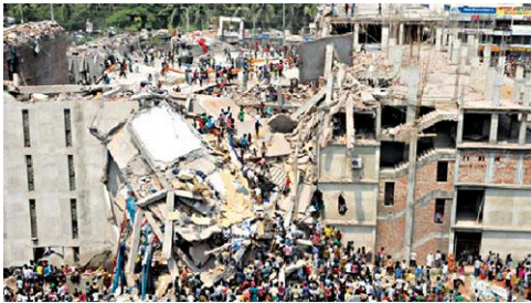
Figure 1: Collapsed Rana Plaza at Savar
